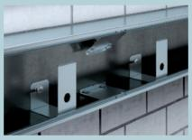
Central alignment using notches
